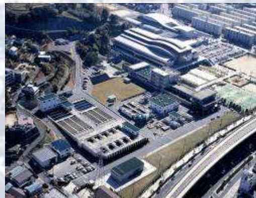
Fig.9 Hiroshima Big Wave and Ushita Filtration Plant
