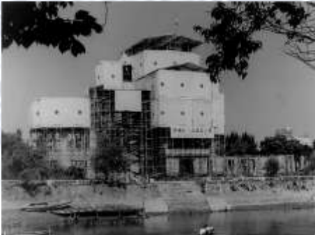
Fig. 10 A-Bomb Dome under first preservation work (1967)
