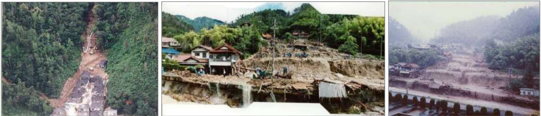
Pictures of landslide damage in the Asaminami and Saeki Wards of Hiroshima City in June 1999.
