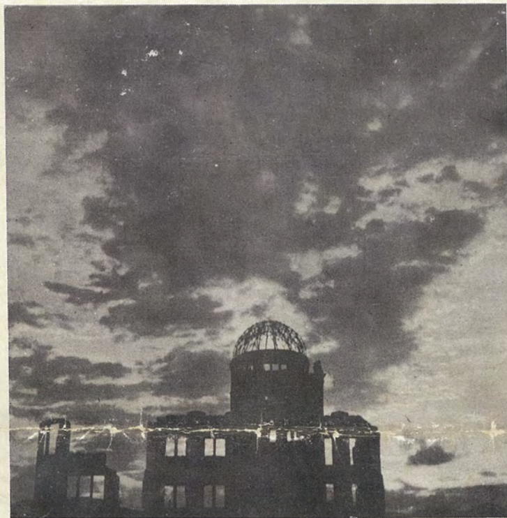
Silhouette of the dome building at the epicenter of the atomic bomb blast.
