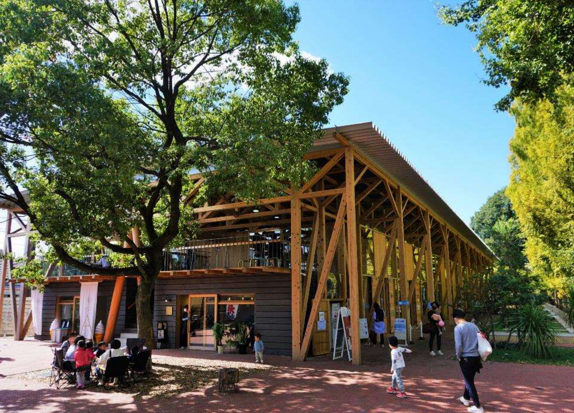
KAKAMIGAHARA BRIDGE PARK (各務原市) 2021.3.27 OPEN
