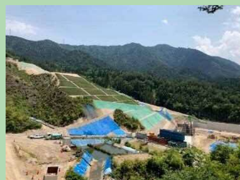
⑥植生基材吹付
