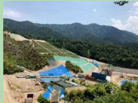
⑥植生基材吹付
